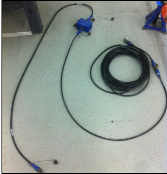
Figure 84 Programming Cables disconnected
