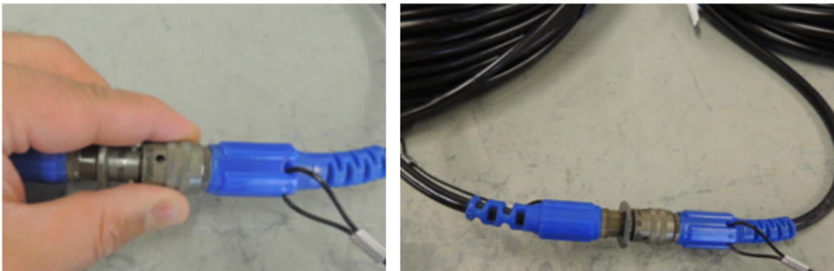
Figure 99 Extension cable 22CABL0033 and Clamp Cable 22CABL0058
