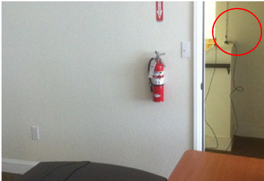
Figure 57 2 x Antenna standing straight outside the structure with the router
