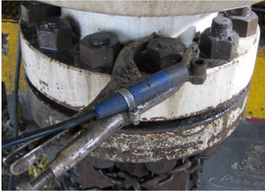
Figure 102 BOP Clamp cable clamp attached to the BOP
